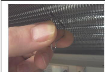
8. Feed the end tip of the sensor bulb into the clip you have just fitted.
