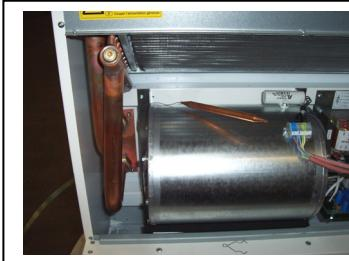
7. Using the spring clips supplied, fit one to the centre of the finned element.
